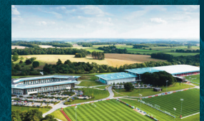
FA National Football Centre at St. George's Park
